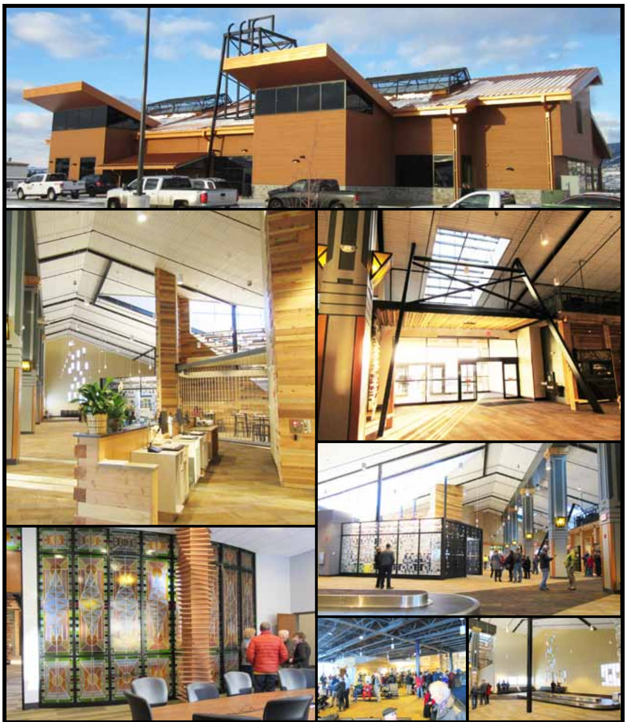
With its open floor plan, high ceilings, skylights and many Butte touches like stained glass and its entrance beneath a towering headframe, the new passenger airport terminal wowed the 300 people who attended its Grand Opening last week. Photos by Robin Jordan
